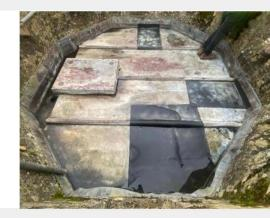
Once the deck was ready to receive the lead, bays were calculated and formed with mop stick hand rail. The lead was cut at ground level, lifted up and laid with skill and care inline with the current code of practice. The lead was welded where necessary and cut into the existing channel in the stone work. Lime mortar specified by the architect was used to point. The lead was then cleaned and coated with patination oil. The finished roof was inspected and approved before striking the scaffold.
