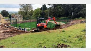
The external perimeter of the site was set out and marked again. A heavy duty weed membrane was laid and Type 1 stone was imported and edgings were installed, land drainage was also installed at this point.
